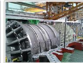
Blade Ring Dismantling, Lifting
