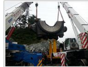
Seating the Exist LP Lower Casing
